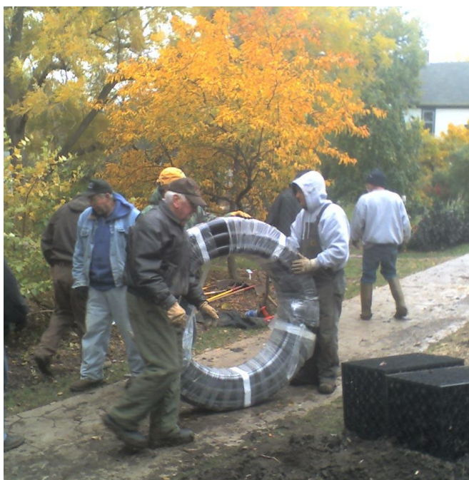
Workers roll out the flexible tubing on the 2 nd day of work at Ward Meade Park. Photo by Don Taliaferro.
