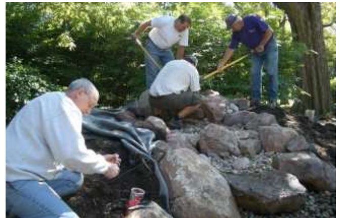
Don Taliaferro, (l-r) Eric Wood, Rob Nordyke and Ray Schroeder work on the new pondless waterfall at Ward Meade Park. Photo submitted by Bob Saathoff.
