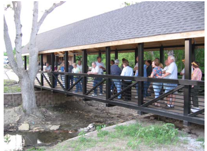
Dave Bartels explains to the group how they are going to build a waterfall coming off the TAWGS pond at Lake Shawnee which will pool under the new bridge.
